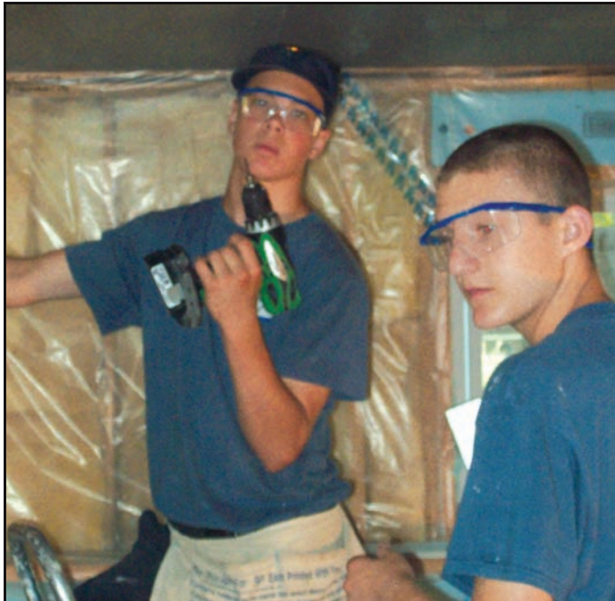
Alex and Gary hang drywall inside the Habitat home.
