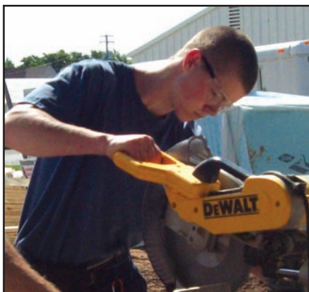
Youth receive valuable work experience using power tools.
